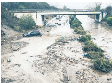
Santa Barbara County Fire Department U.S. Highway 101 at the Olive Mill Road overpass is flooded with runoff water from Montecito Creek on Tuesday in Montecito, Calif.
